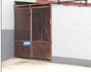
Photo of the sanitary facilities Hazardous waste storage area.JPG
