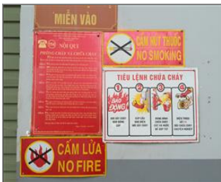
Photo of fire safety equipment Fire warning sign.JPG
