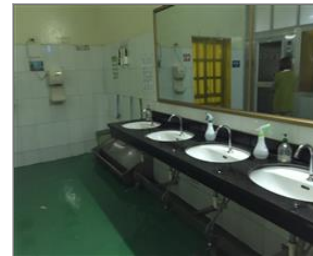
Photo of the sanitary facilities Hand washing area.JPG
